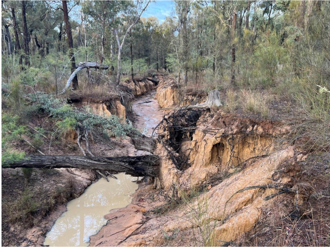
Creek erosion from early logging
