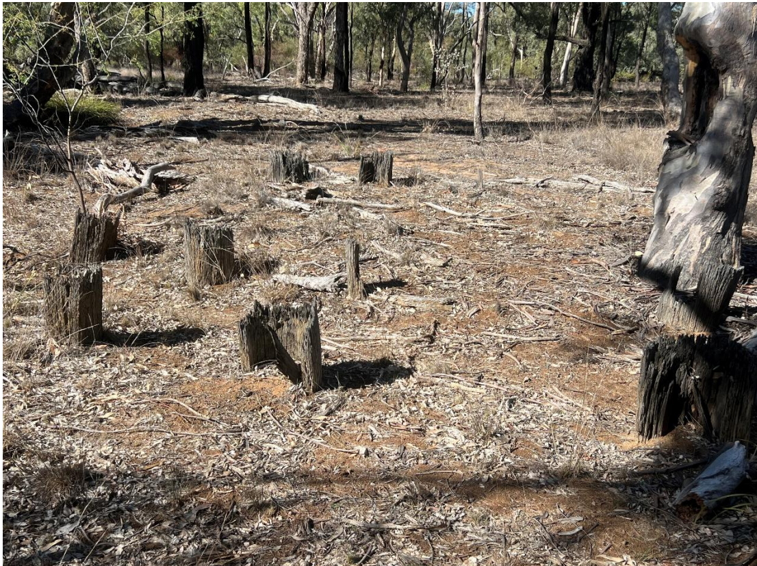
Foundation stumps of late 19 th C inn at sleeper cutters camp, Three Corners Waterhole
