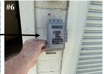
To access button, lift the lid using the black-colored tab as indicated in photo.
