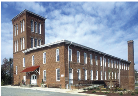
Prizery/R.J. Reynolds Tobacco Warehouse, South Boston, Virginia (1900). Rehabilitated for commercial use. Photographs: Ian Bradshaw.
