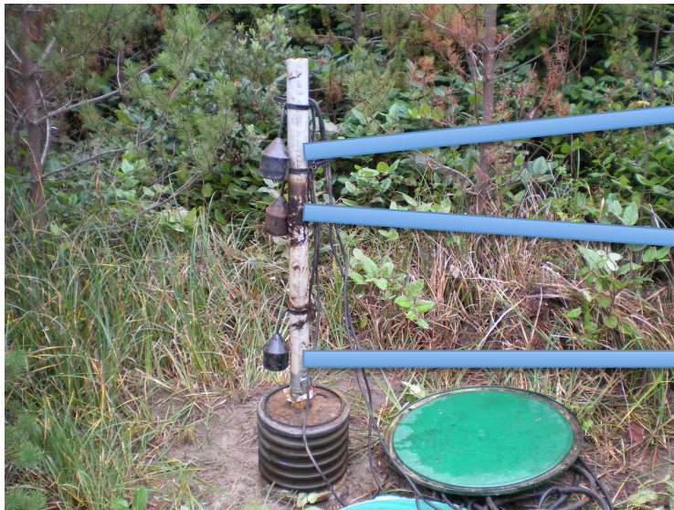
Pump control box with alarm light. Alarm lights up if top float goes on; indicating pump failed to lower water level.
