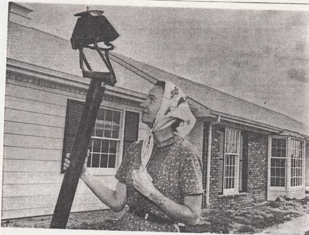
A bent iron lamppost is all that stands as a reminder of the Jan. 24 tornado that leveled the Richard Snyder home in River Bend Estates in Chesterfield. The neighbors were so kind during the 10 days Mrs. Snyder was hospitalized following the tornado that the Snyders told the contractor they wouldn't consider moving away. Their new house will be ready next week.
