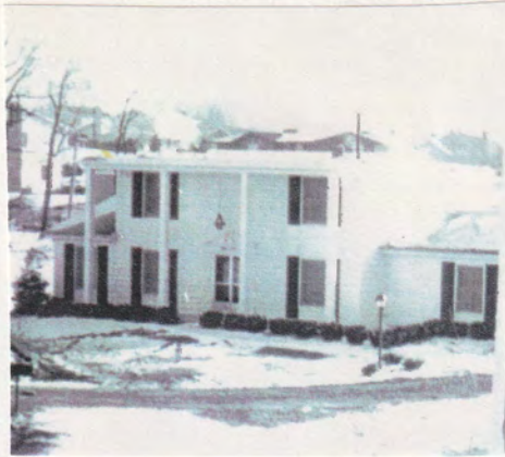
168 Southdown - It used to have a roof!
