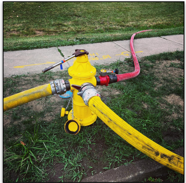
Heavy Hookup - Dual 4" Feeds Going to the Engine Side Intakes, and additional 2-1/2" Feed
