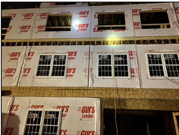
Exterior view of Type 5 Floor and Roof Truss Lightweight Wood Frame Apartment Building
