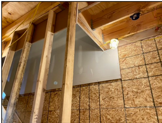
Partially constructed open stairwell with OSB backer that will be behind finished drywall
