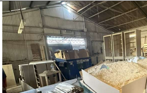
No exit sign (Rear)
