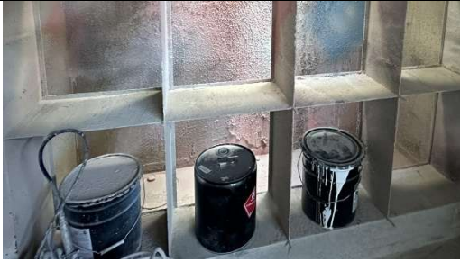
Flammable liquids stored in spray booth
