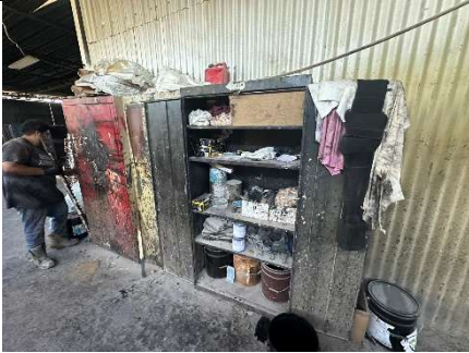
Improper flammable storage
