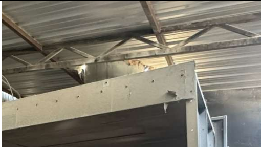
Spray Booth Ceiling Openings
