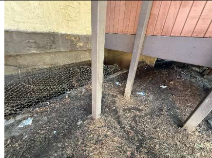
Exposed crawl space
