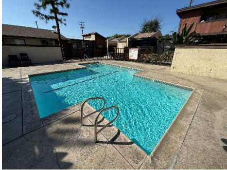
Missing depth markers
