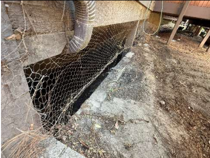
Exposed crawl space
