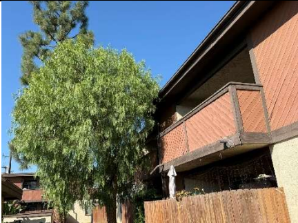
Tree touching building
