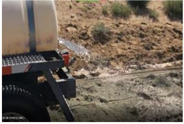
CBR: .1 penetration, up to 2,600 psi, it is hydrophobic, anionic, Rapid set time, in situ mix or pump, full traffic 8 to 12 hrs.
