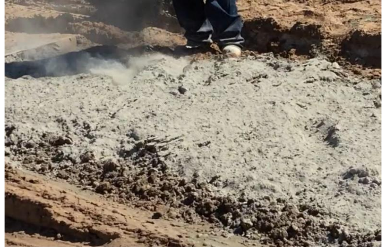
CBR: .1 penetration, up to 1,925 psi, it is hydrophobic, anionic, Rapid set time, in situ mix or pump, full traffic 8 to 12 hrs.
