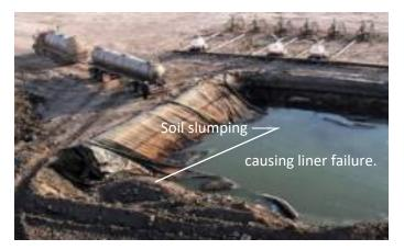
(Above) Pond Liner failure due to slumping soil from recent rains. This could have been avoided with Pro-Sea*IECCO* System<sup>®</sup> O stabilization under the liner. Table (below) displays the results of Atterberg Limit and Plasticity testing for natural wet soils mixed with the Pro-Sea*IECCO*<sup>®</sup> Stabilization System containing >16% minimum +4% Moisture Content (MC).
