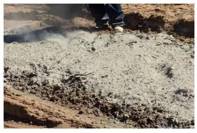
CBR: .1 penetration, up to 1,925 psi, it is hydrophobic, anionic, Rapid set time, in situ mix or pump, full traffic 8 to 12 hrs.
