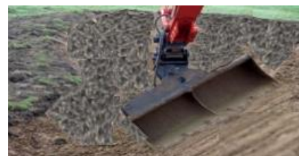
Back drag for light compression.
