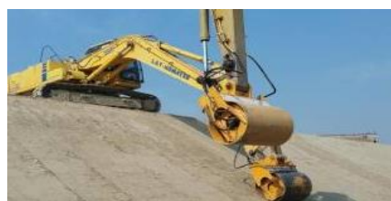
Drum roll for tight compression.
