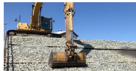
Spread specified rock screen line.
