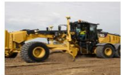
6. Re-grade To Slope and Drain as needed
