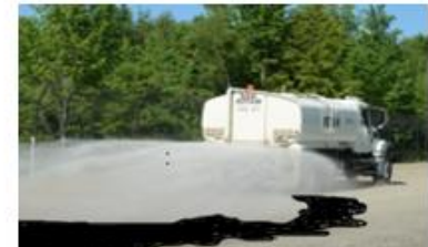
11. Spread Pro-SealECCO FlexSystem II Primary Containment Barrier
