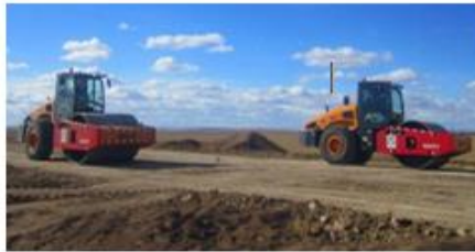
8. Drum Roll Flats and Slopes for Deep Compression
