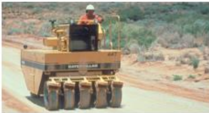
9. Pneumatic Roll for Surface Densifying Compression
