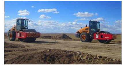
5.a Drum roll flats for deep compression
