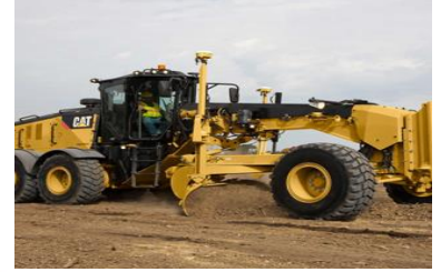
1. Grade To Slope and Drain
