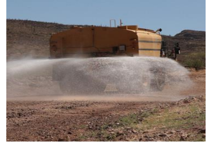
3. Wet To spec'd Moisture Content
