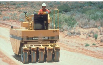
9. Pneumatic Roll for Surface Densifying Compression
