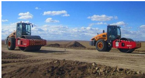
8. Drum Roll Flats and Slopes for Deep Compression
