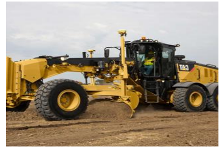
6. Re-grade To Slope and Drain as needed
