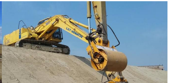
8. Drum Roll Flats and Slopes for Deep Compression
