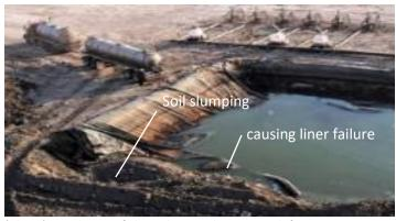
(Above) Pond Liner failure due to slumping soil from recent rains. Avoided this use Pro-Sea/ECCO System® O stabilization under the liner.
