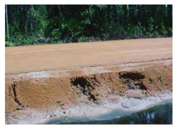
(Above) this road base is placed in extreme wet environs. Table (below) displays the results of Atterberg Limit and Plasticity testing for natural wet soils mixed with the Pro-Seal ECCO® Stabilization System containing >16% minimum +4% Moisture Content (MC).
