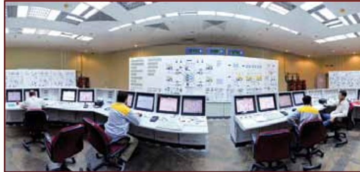
Iranian operators monitor the nuclear power plant unit in Bushehr, about 1,215 km (755 miles) south of Tehran
