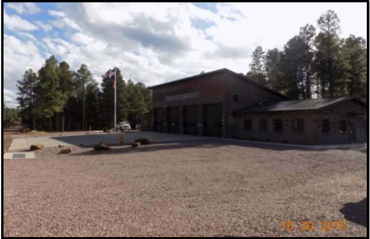
New Fire Station as Viewed from Merzville Road (October 30, 2018)
