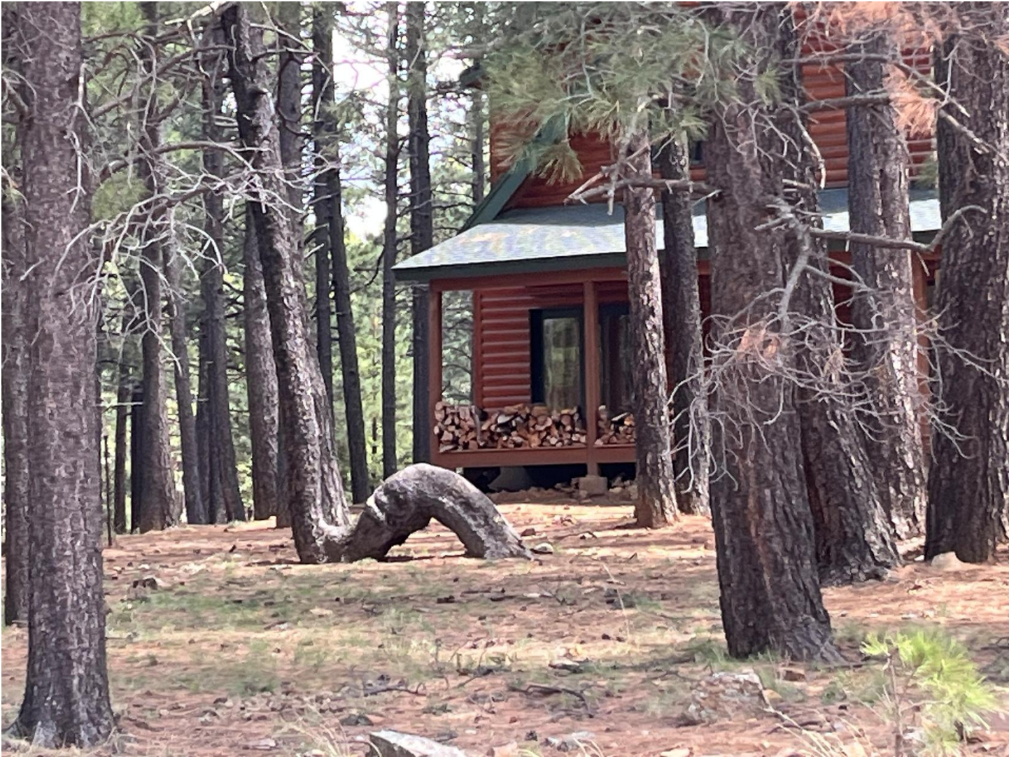
Firewood on deck. Needle layer on asphalt shingle roof.
