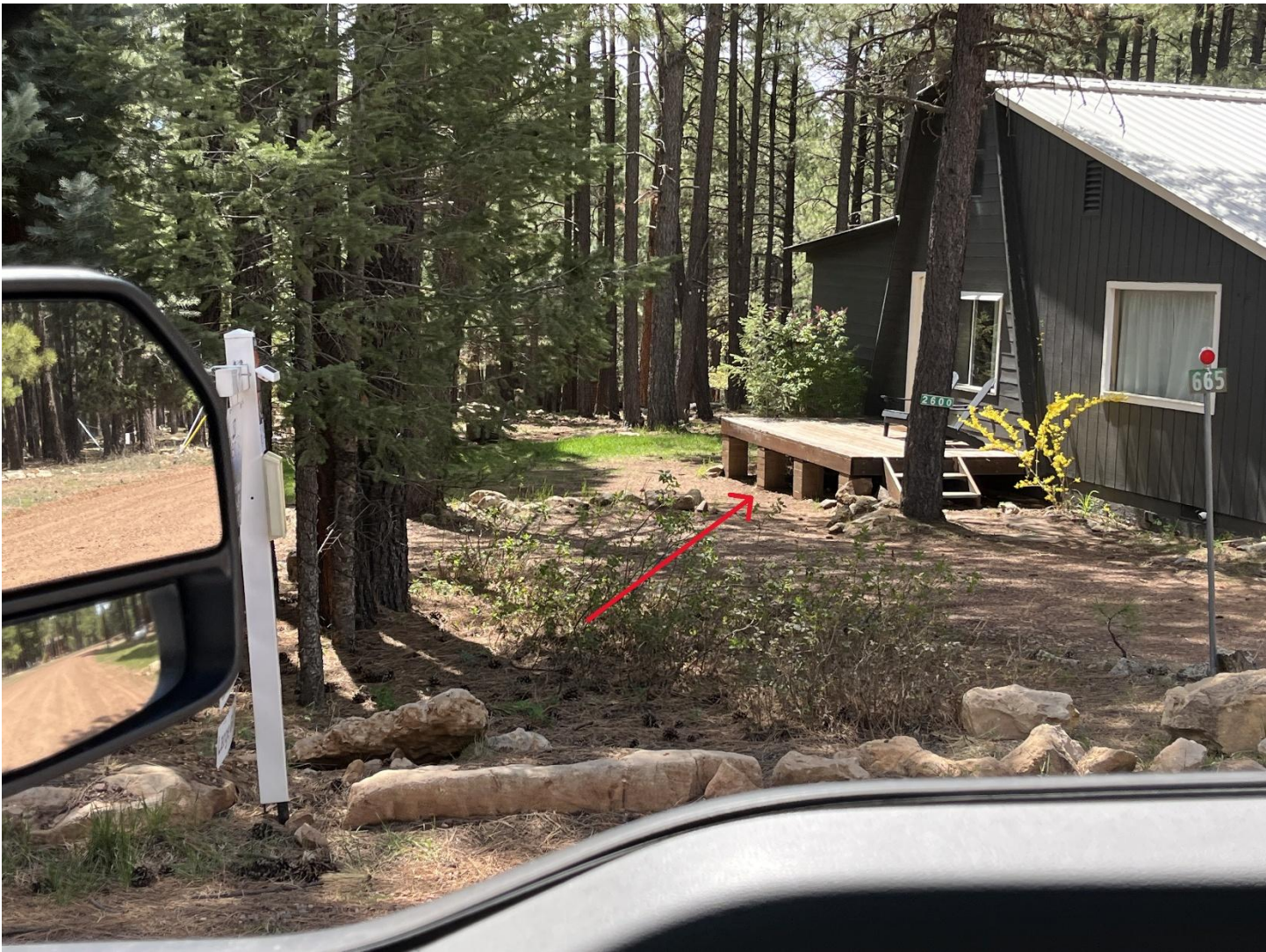
RED arrow identifies good bare dirt within the immediate zone (0-5ft) from wooden deck.
