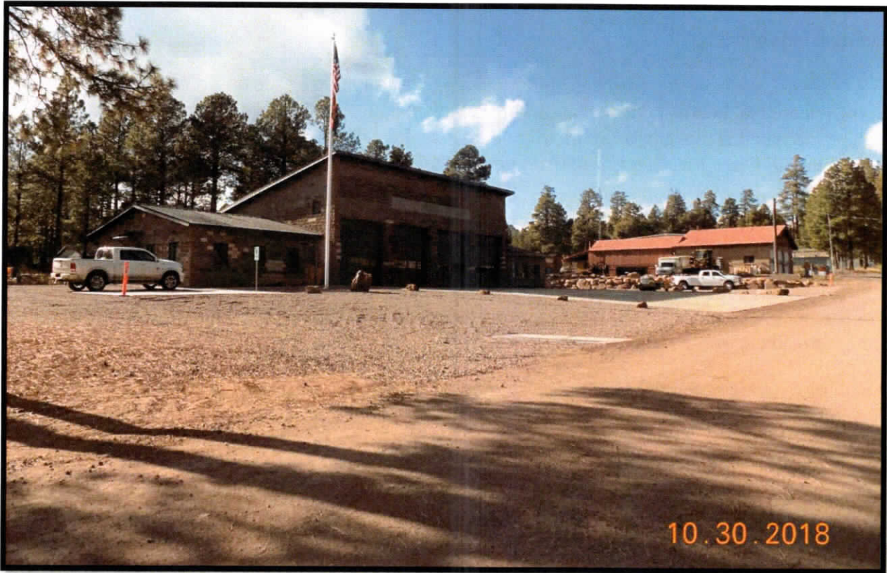
New Fire Station and Annex as Viewed from Merzville Road (October 30, 2018)
