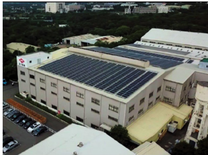
Rooftop Mounting PV System
