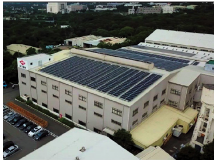
Rooftop Mounting PV System
