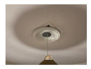
Notes: Gap between light fixture and wall. Recommend patching and repairing.
