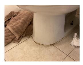
**Notes:** Recommend caulking around toilet to prevent water from entering underneath floor/subfloor.
