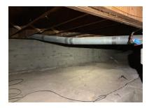
Note: In the crawl space, I discovered duct tape around one of the ducts.
