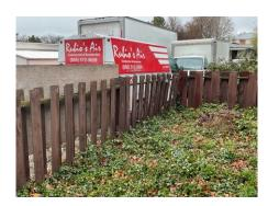
**Note:** Various parts of the fencing is sagging towards the home. Recommend further evaluation by a fencing contractor to see if the fence can be fixed and also stained to extend the life of the fence. Some locations appear to be warped and may not be salvaged.
