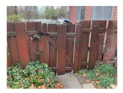
**Notes:** Missing hardware. You need to lift the gate up and open as to not hit the concrete. Hinges need to be adjusted.
