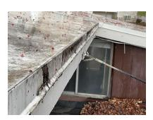
**Notes:** Between not having gutters installed and the vegetation from the nearby tree, this is causing mildew buildup. Recommend further evaluation by roofing contractor to install gutters and downspouts to help protect the fascia.
