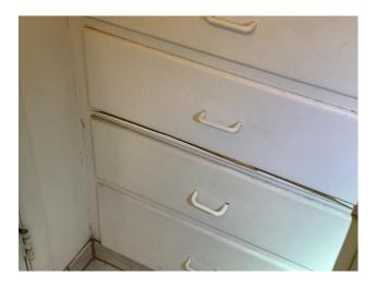
**Notes:** Cabinet drawer behind bathroom door is cracked. Some cabinets are hard to open and or do not close properly.
