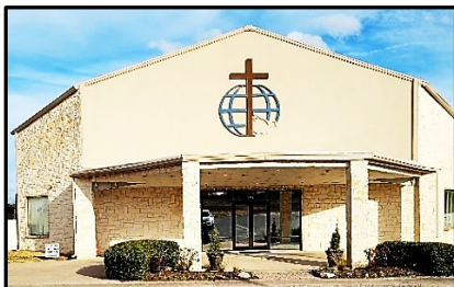
Same church two years after cleaning with Nano cleaner then sealed with Stayz Sealer™
