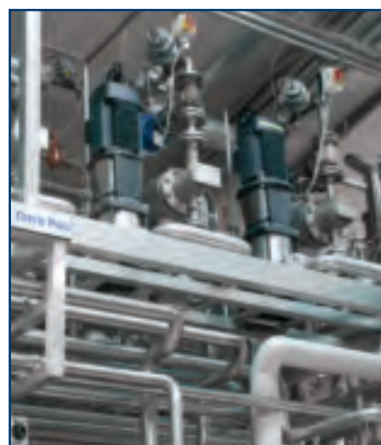
CR pumps installed in a dairy plant
