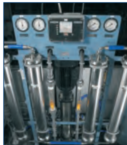
CRN 5 installed in a water treatment plant
