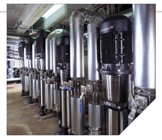
and do not require any additional tank to provide supplementary pressure. In boiler feed applications, where many big tanks are gathered, a compact system is an advantage.
