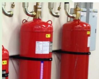
**Wall Bracket:** To fix the cylinder to avoid any vibration during activation process.
