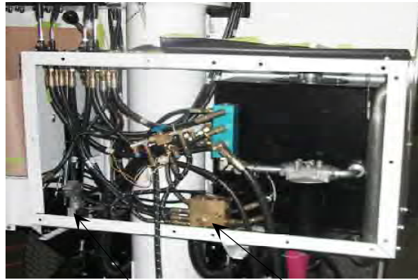
Hand Pump Check Valve Manifold
