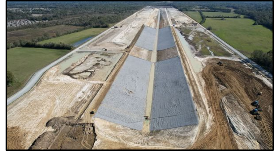
Construction Underway for Comite River Diversion
