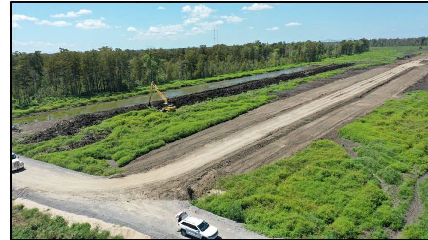
Construction Underway for Westshore Lake
