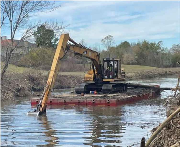
FIGURE 2-53: CLEARING AND SNAGGING OF BASIN WATERWAYS (PHOTO SOURCE: USACE)
