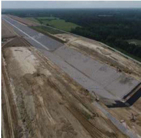
CHANNEL SEGMENT 2A, 90% COMPLETE (PHOTO SOURCE: USACE)
