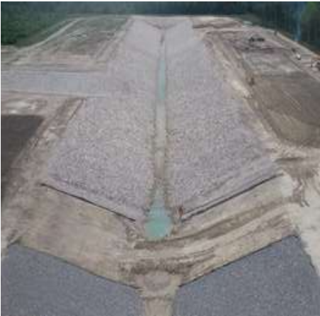
CYPRESS BAYOU, 80% COMPLETE (PHOTO SOURCE: USACE)
