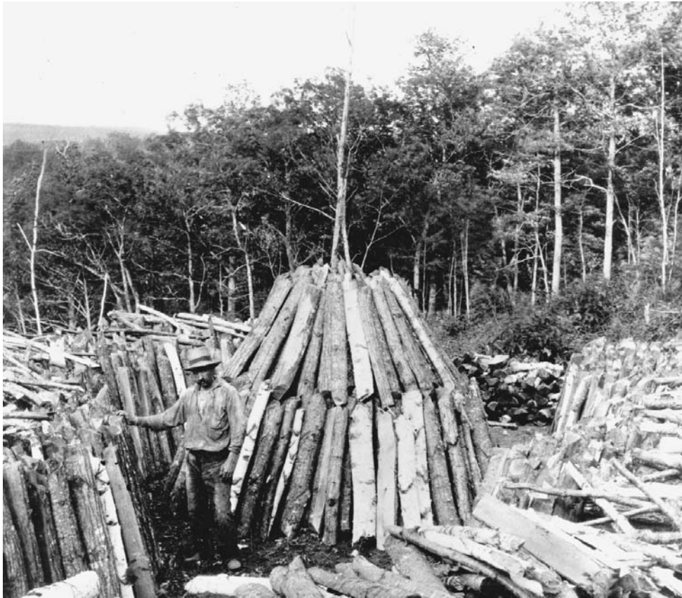
Figure 5. Charcoal making in 1900 using methods unchanged for centuries. The wood is stacked in the shape of a cone, covered with earth, and then ignited and carefully tended.
