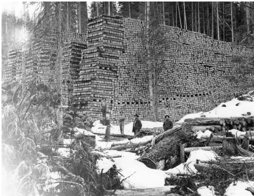
Figure 9. Railroad bridges and trestles (top) were constructed of pilings and large timbers. Railroads consumed vast quantities of wood, as these stacked cross-ties show (bottom).
