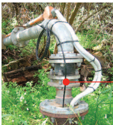
Gunmetal wafer type valve mounted between flanges
