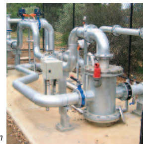
Submersible pump installation
