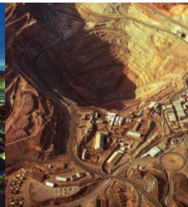
Dust suppression and slurry pumping facilitated by water flow controlled with Maric Valves
