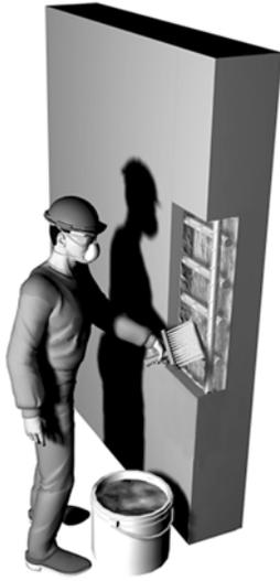
Fig. 6—Treatment of exposed reinforcement.
