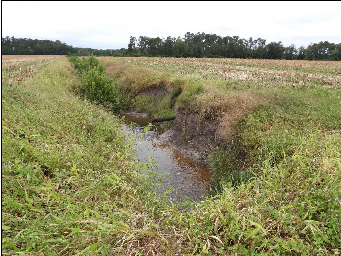
Figure 13. Image of central ditch on site (looking east) revealing a 7' drop and an exposed drain tile outfall. Image by Michael J. McGraw at Linkhaw Farms on September 23, 2023.
