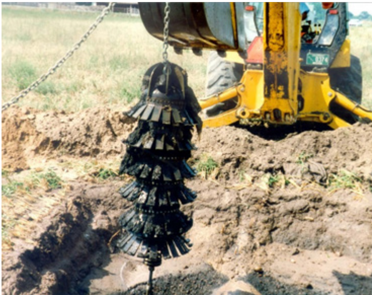
Pipes are cleaned with drag scrapers that correlate with pipe size.
