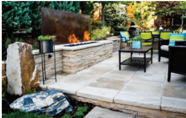
Above: this house in a suburban setting sits on a sloped hillside with other houses looking into its back yard. Ecoscape was hired to create an intimate outdoor space that would address drainage mitigation and privacy issues. This small, 20' X 12' outdoor room is packed with features that compliment each other. A gas fireplace set off by placing a rusted metal panel behind it is a major focal point from inside the house. Soft buff flagstone patio and walls contrast with the fireplace and a black quartz pyramidal water feature close to the house, which is echoed by large natural boulders at left front. 'Moon Glow' junipers behind the fire and a "forest planting" of evergreen and deciduous trees separate the patio from the driveway.
