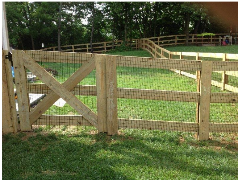
Picture 1 – Kentucky 3 Board Fence Example
