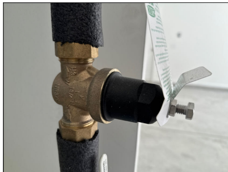
Pressure reducing valve (PRV)
