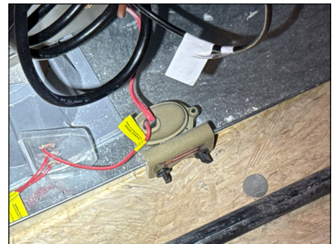
Condensate overflow switch noted
