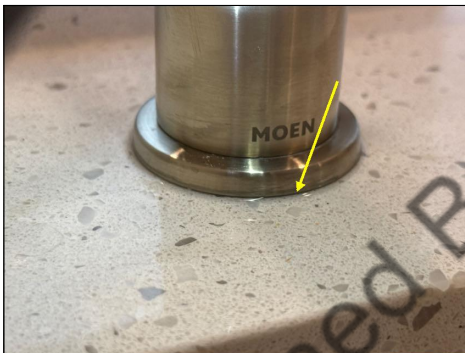
Leaking Faucet - Left Master Sink
