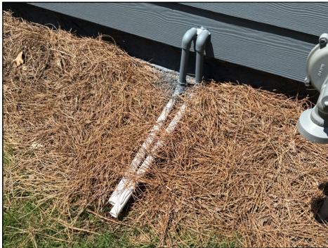
Condensate drain pipe
