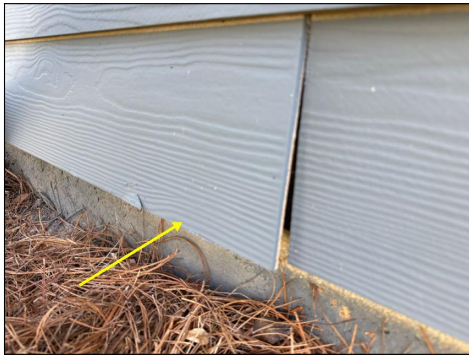
Loose Siding - Left Side
