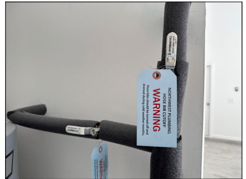
Hose bib shut off valves - Garage
