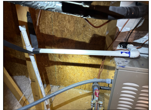
Condensate drain pipe
