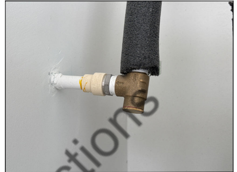
Vacuum Relief Valve (VRV)
