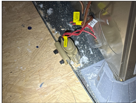
Condensate overflow switch noted
