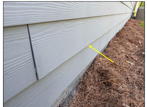
Loose Siding - Left Side
