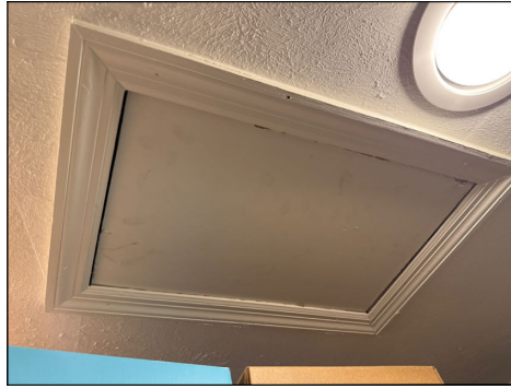
Recommend Weatherstripping/insulation - Master Closet
