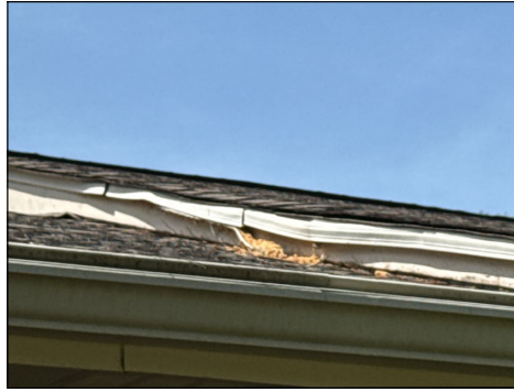
Damaged Drip Edge - Left Side
