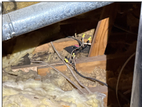
Wires Outside of Junction Box
