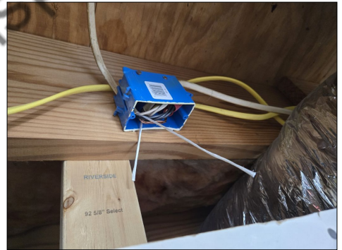
Open Junction Box - Basement Hall Closet
