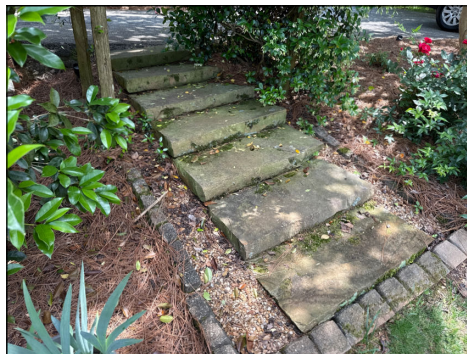
Missing Graspable Handrail - Left Side Stairs
