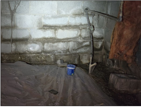
Efflorescence - Front Left Corner
