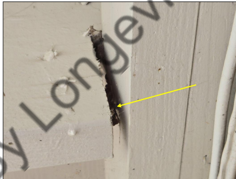
Separating Deck Joist - Rear Deck
