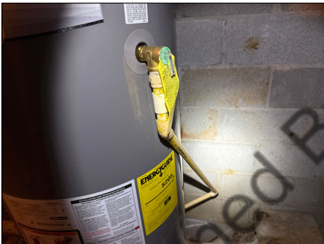
Improper TPR Install
