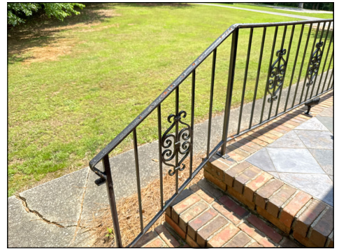
Loose Handrail - Front Porch
