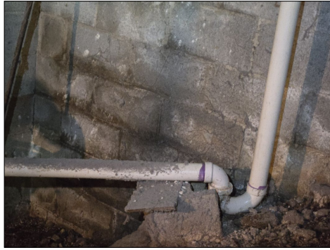
Efflorescence - Front Right Corner
