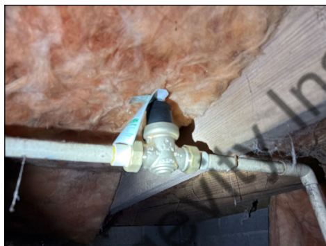
Pressure reducing valve (PRV)
