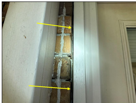
Gap - Rear Basement Right Door
