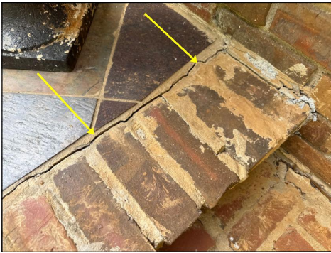
Re-point/repair grout - Front Porch
