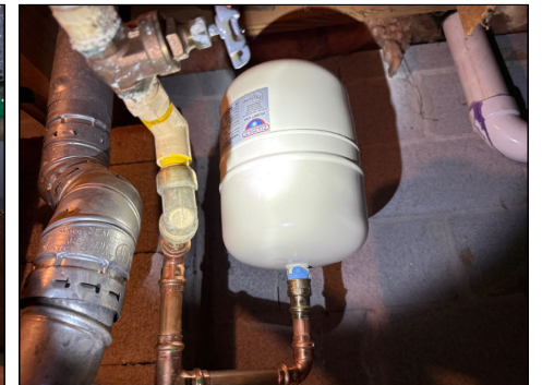
Thermal expansion tank
