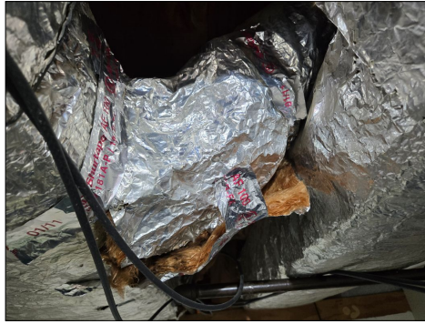
Torn/Damaged Ductwork - Crawlspace
