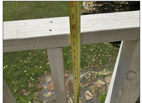
Improper Guardrail Height - Rear Deck
