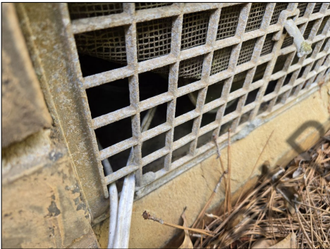
Damaged/Missing Screen(s) - Front Side
