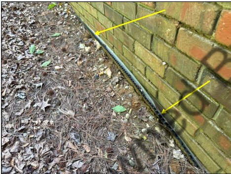
Exposed Waterproofing Material - Right Side
