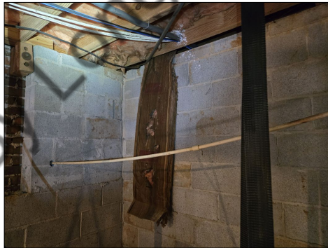
Loose Insulation - Crawlspace
