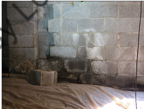
Efflorescence/Possible Moisture Intrusion - Left Rear Side
