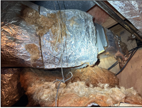
Torn/Damaged Ductwork - Crawlspace
