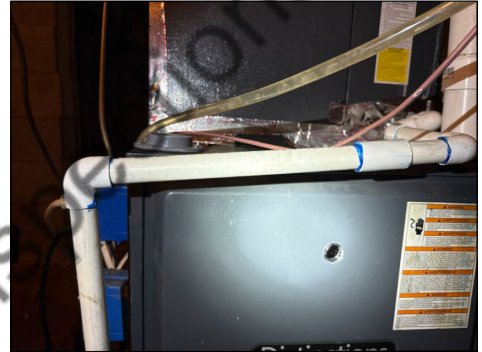
Condensate drain pipe
