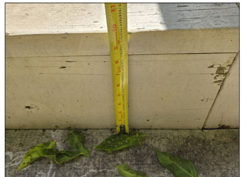
Improper Stair Riser - Rear Deck Stair
