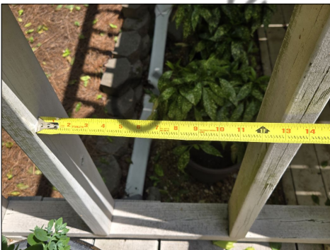
Improper Vertical Picket Width - Rear Deck
