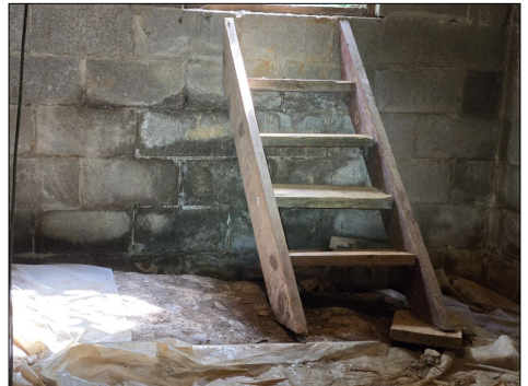
Efflorescence/Possible Moisture Intrusion - Left Rear Side
