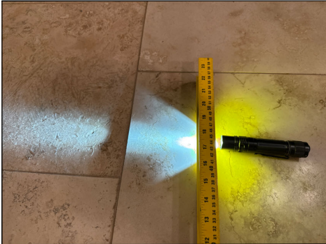
Uneven Floor(s) - Master Bathroom
