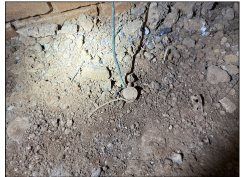
Ground wire and rod noted.
