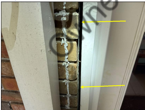
Gap - Rear Basement Right Door
