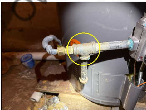
Improper T Fitting
