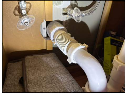
Flex Pipe - Left Master Sink
