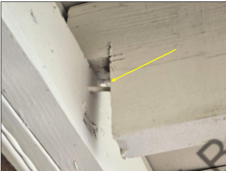
Separating Deck Joist - Rear Deck
