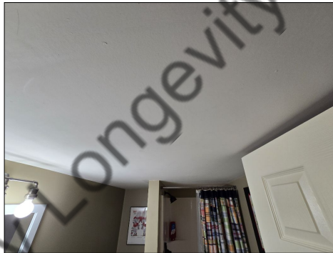
Missing Fan/Window - Basement Bathroom
