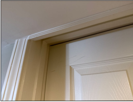
Conflict with Door Jamb - Front Right Basement Hallway Door
