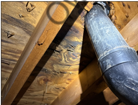
Moisture Stain - Right Side Vent Stack
