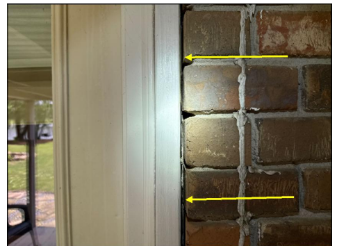
Gap - Rear Basement Right Door
