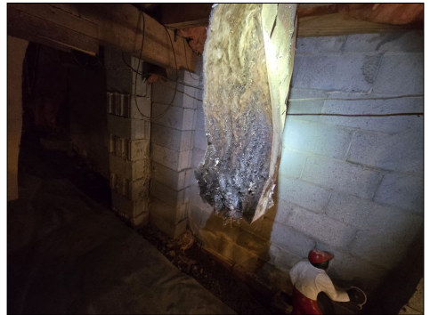
Suspect Fungal Growth/Loose Insulation - Crawlspace
