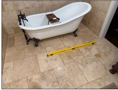
Uneven Floor(s) - Master Bathroom
