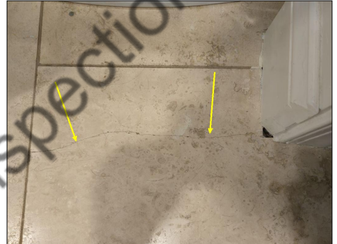
Cracked Tile - Master Bathroom
