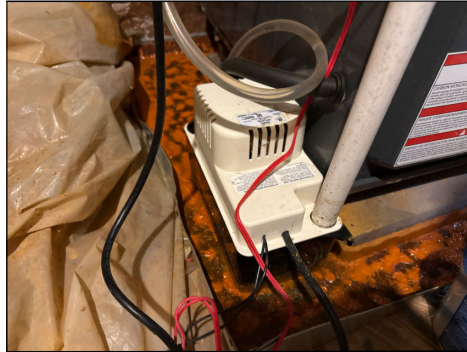
Condensate drain pump noted
