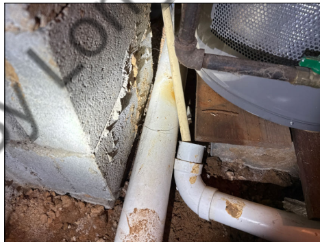
Improper TPR Install
