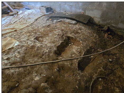
Missing Vapor Barrier
