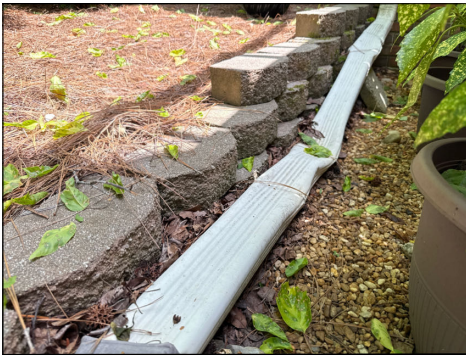
Damaged Downspout - Rear Side
