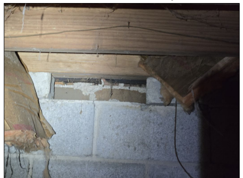
Blocked Vent - Rear Side of Crawlspace
