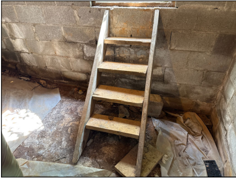
Loose/Not Attached Properly - Crawlspace Stairs
