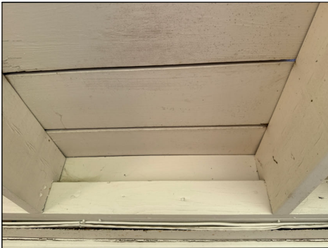
Missing Flashing - Rear Deck
