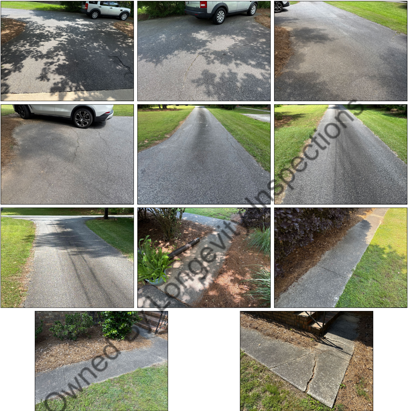
Damaged Concrete - Sidewalk
