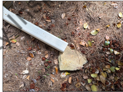
Missing Splash Block - Rear Side
