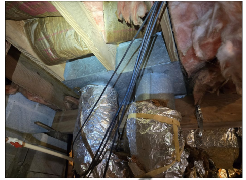
Missing Insulation - Crawlspace
