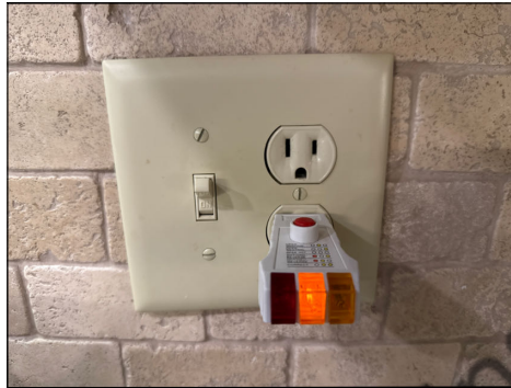
Open Ground - Right of Kitchen Sink
