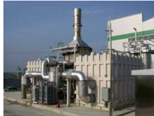
UC San Diego's 2.8-megawatt fuel cell is being manufactured by FuelCell Energy, Inc. UC San Diego's Energy Innovation Park has a compressed natural gas fueling station for campus vehicles.
