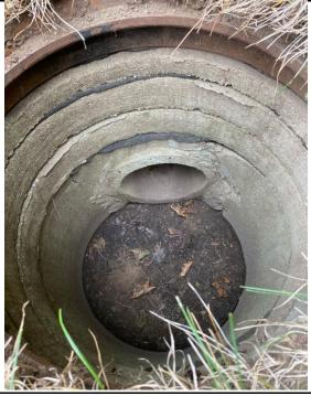
Catch Basin #25 backyard of 48 Talcott. Dry sediment 3 inches below invert. Approx 13 inches sediment at thickest point.
