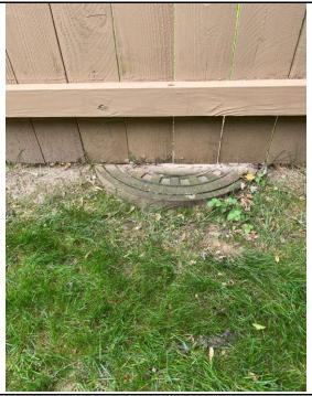
**Subject** Manhole #7, along 44/46 Talcott. Fence owned by 44 Talcott constructed over manhole.
