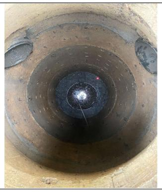
Subject Dry Well #4 in detention basin. Visible to bottom. Minimal/no siltation.
