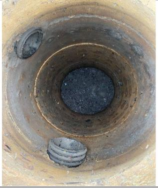
Subject Dry Well #7 in detention basin. Dry silt at bottom of well, approx 6 inches sediment.
