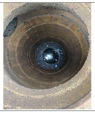
Subject Dry Well #3 in detention basin. Visible to bottom. Minimal/no siltation.
