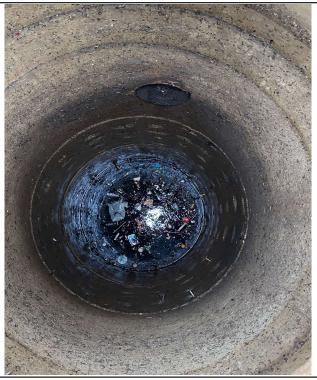
Subject Dry Well #9 in detention basin. Bottom of well under approx 6 feet water. Floating debris.
