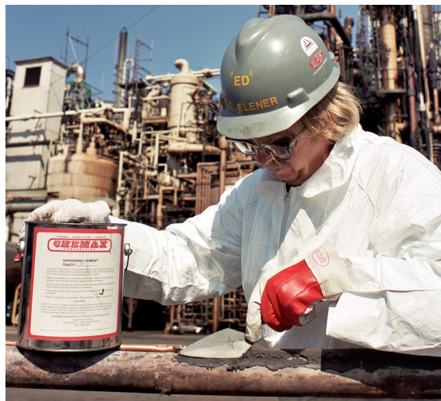
Figure 1: Typical Steam Tracing Application
