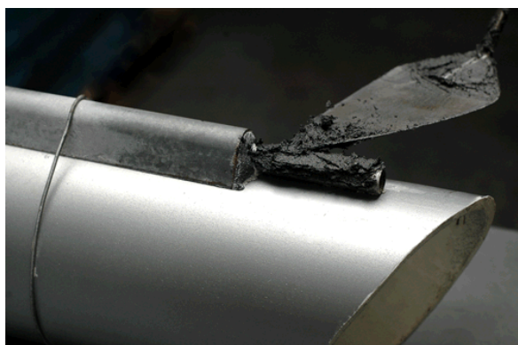
Figure 2: Mastic Being Applied to Bare Tracer
