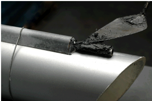
Figure 2: Mastic Being Applied to Bare Tracer
