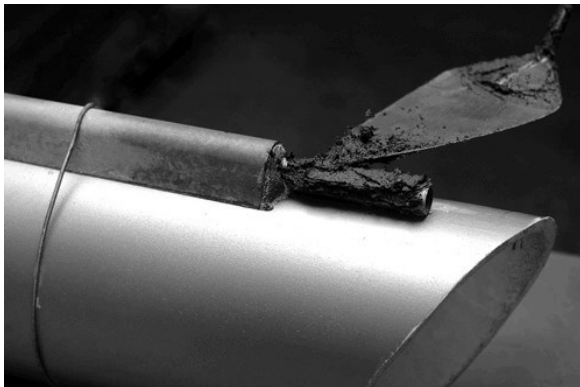
Figure 2: Mastic being applied to bare tracer
