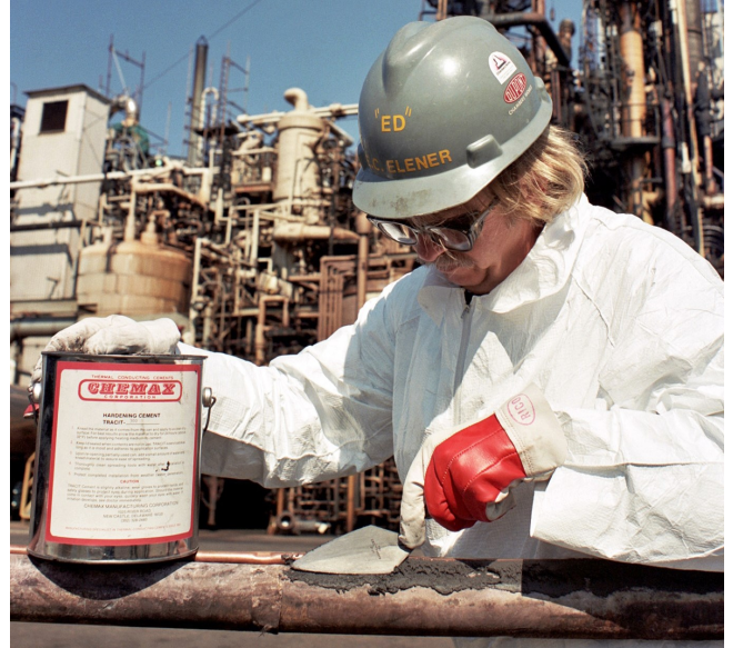
Figure 1: Typical Heat Tracing Application
