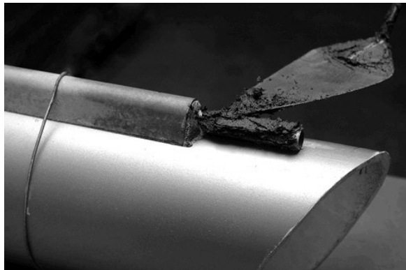
Figure 2: Tracit being applied to bare tracer.
