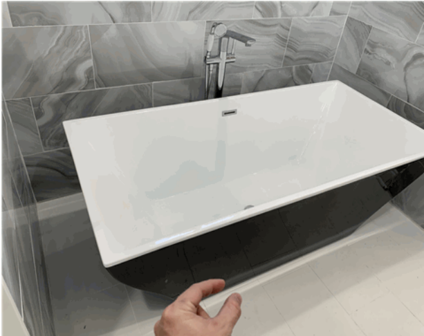
Tub moves when leaning over tub to turn on water
