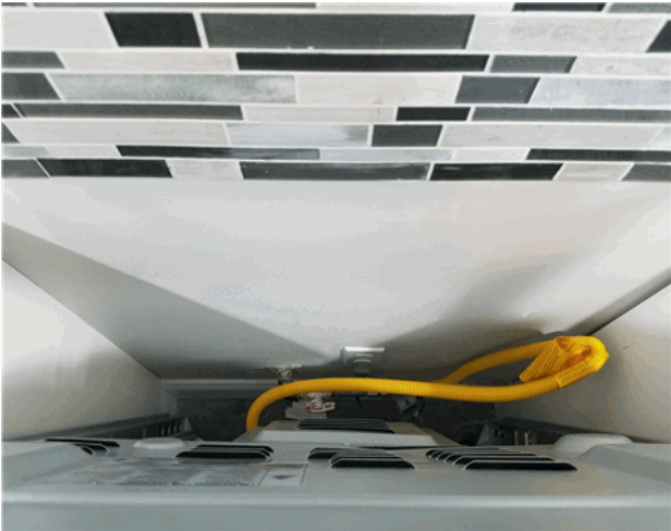
Anti-tip bracket was missing @ range. Install to prevent tipping
