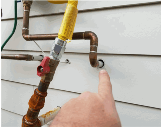
Seal openings @ water heater
