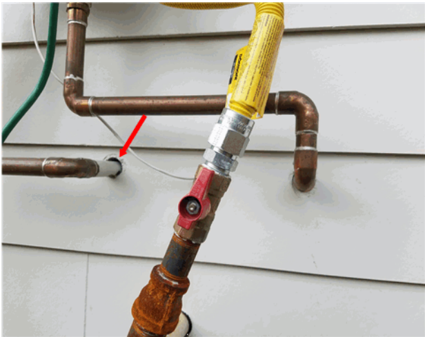
Seal openings @ water heater
