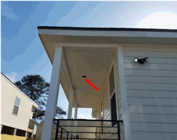
Install missing can trim @ back patio
