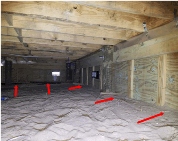
Wood to ground contact
