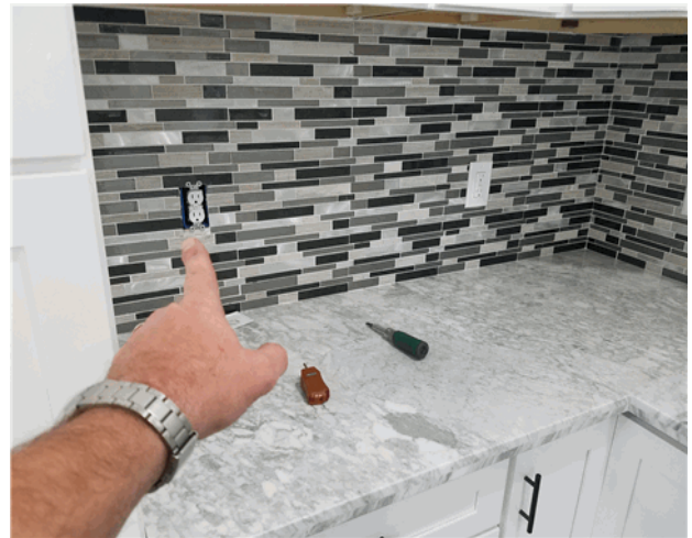
Loose outlet - secure - install outlet cover plate (damaged)
