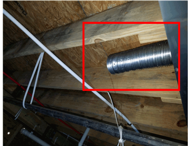
Dryer vent open under home - back-center
