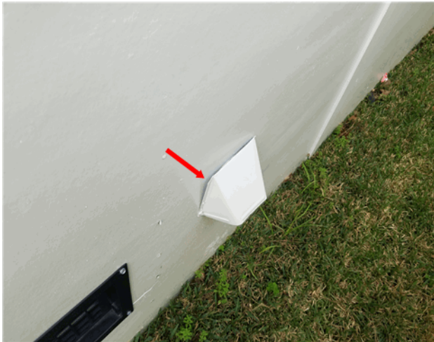
Secure dryer vent and seal
