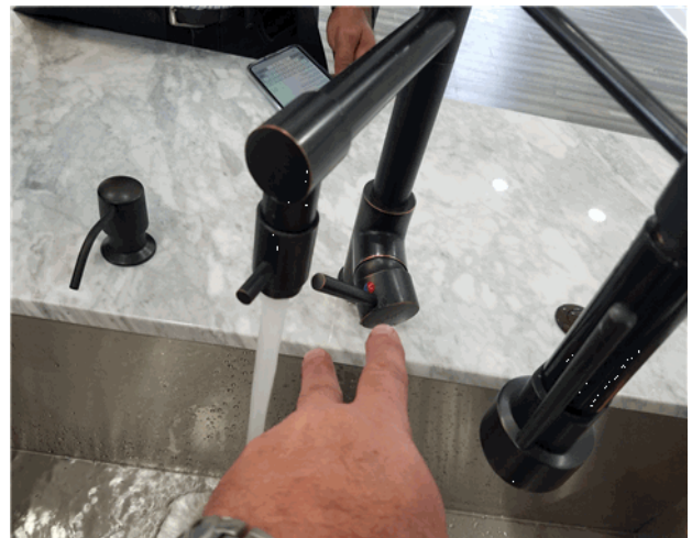
Adjust fixture handle to right side
