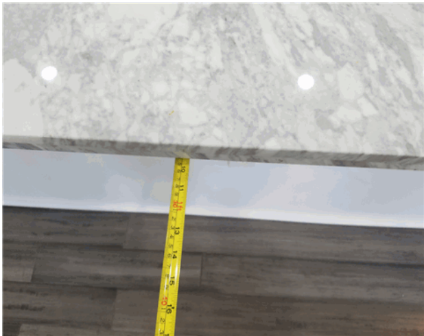
Counter-top extend out pass cabinet by 9.5 inches
