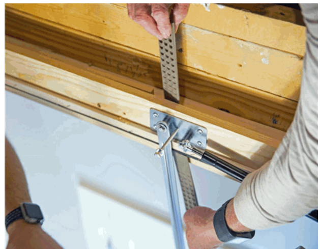
How to use and install shims
