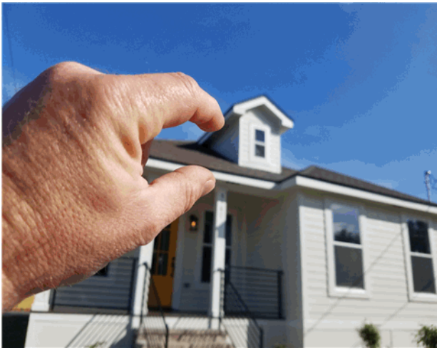
Improper clearance @ dormer siding and shingles.
