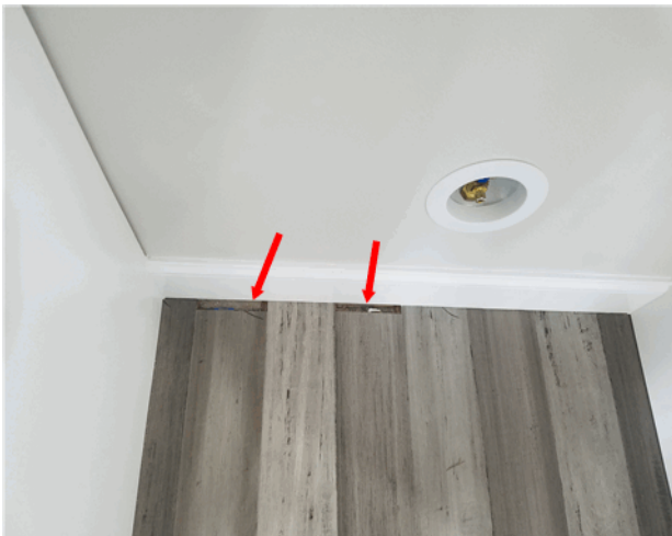
Small gaps @ interior kitchen floor - refrigerator area
