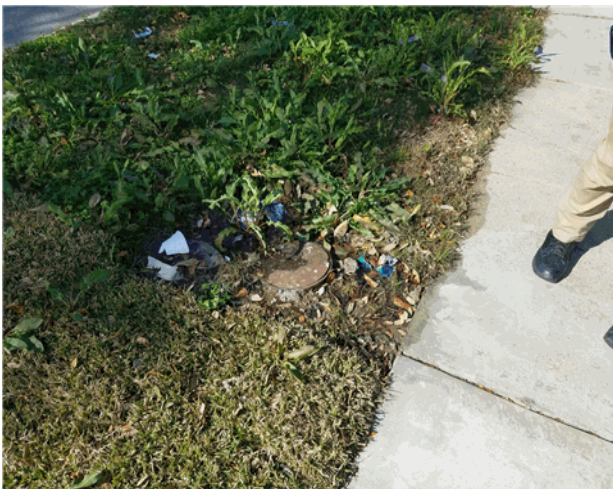
City Connection @ street - leaking
